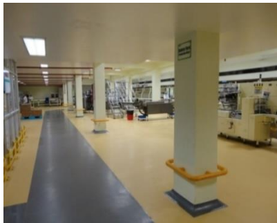
Fig 4- Wall and pillar guards used to avoid daily wear and tear of the surfaces
