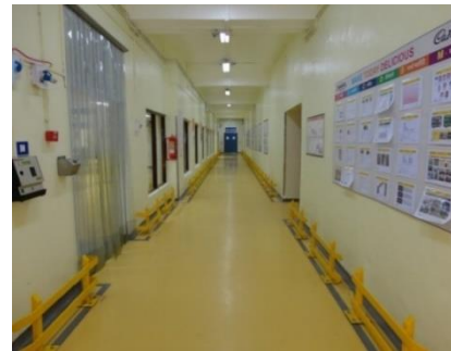
Fig 4- Wall and pillar guards used to avoid daily wear and tear of the surfaces
